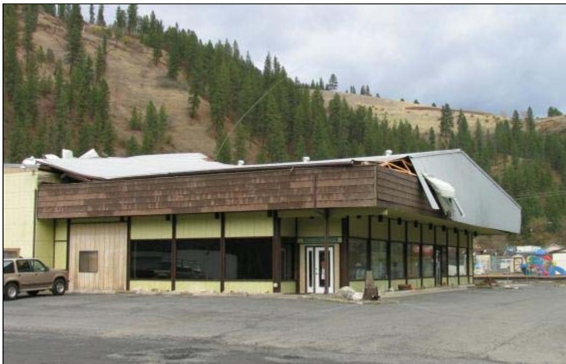
**This photo shows how much the pitched roof moved during the storm.**
