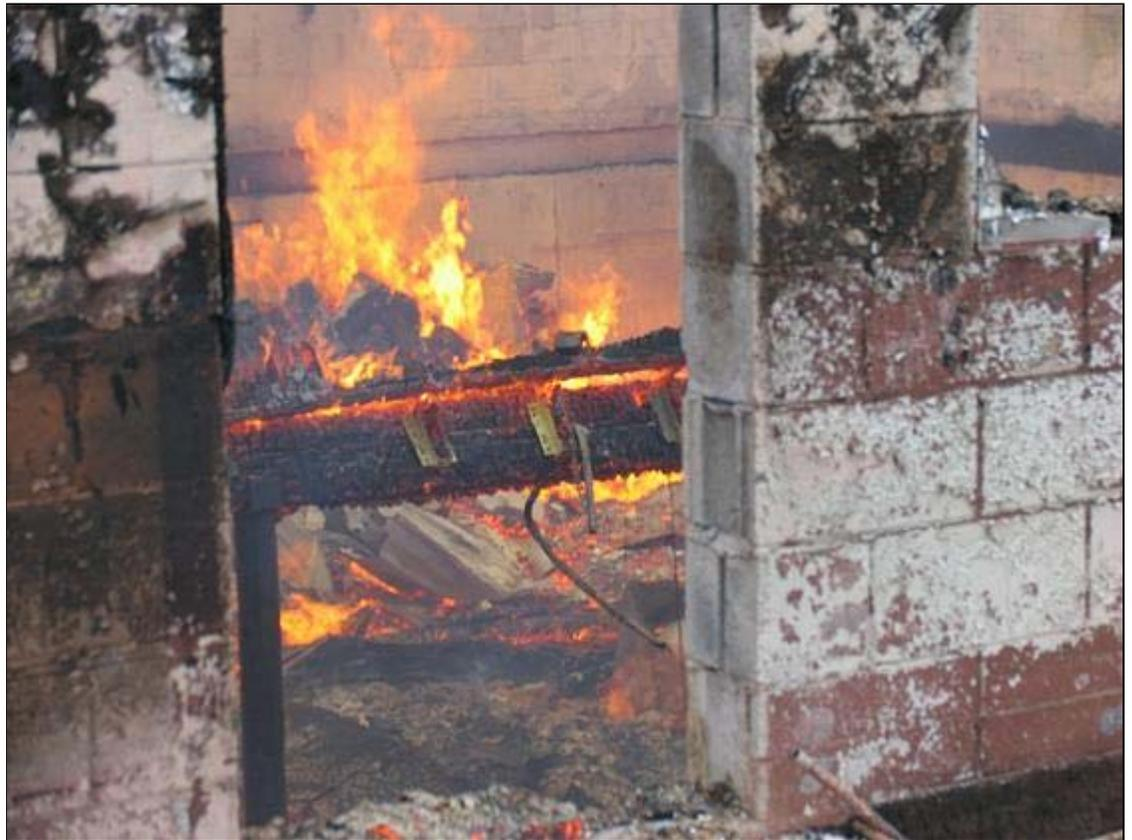
Flames have burned through the flooring and the basement is opened to view.
