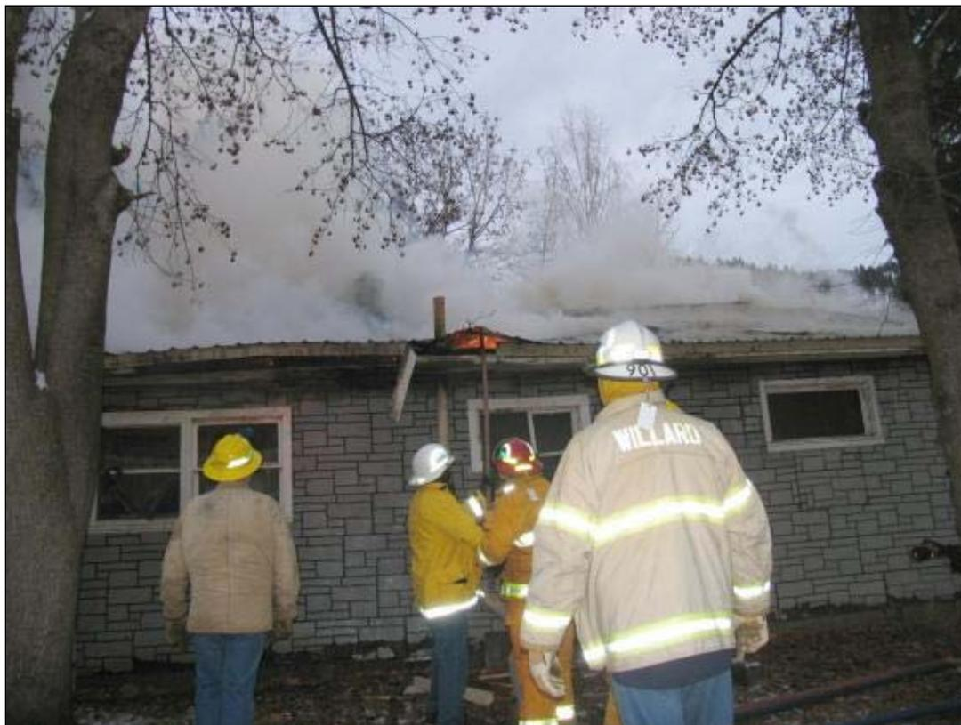
Fire fighters work to open up access to the area between the roofs so they can better fight the blaze. Three roofs and three ceilings made reaching the fire difficult.
