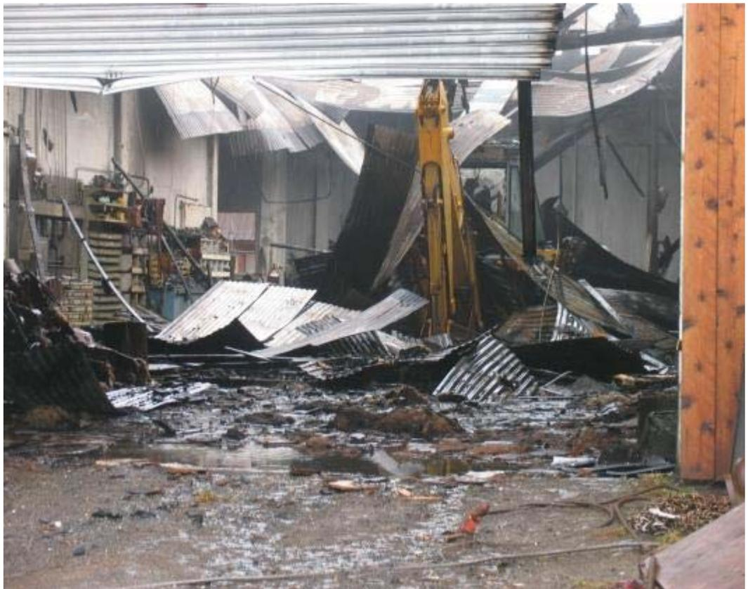
**Collapsed roofing materials are on this backhoe that was damaged in the fire.**
