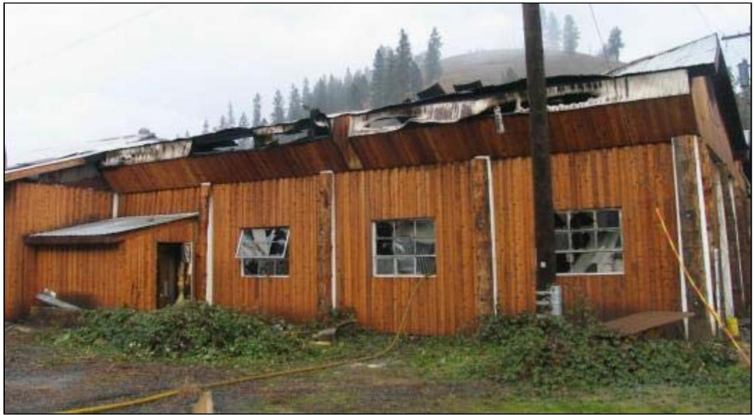
A view of the damage from the back of the shop shows collapsed portions of the roof.
