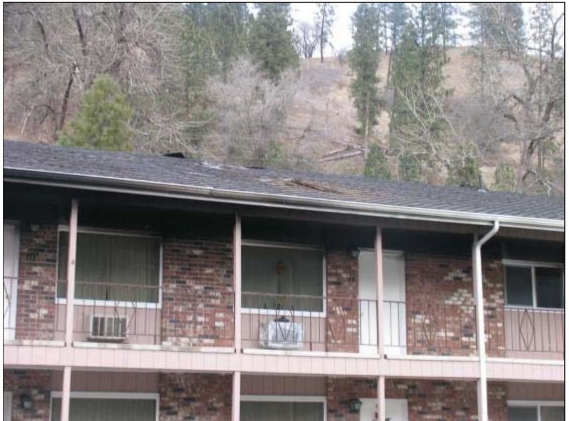
The roof shows evidence of where fighters made a trench cut in the roof of this apartment to make sure there was no fire in the attic.
